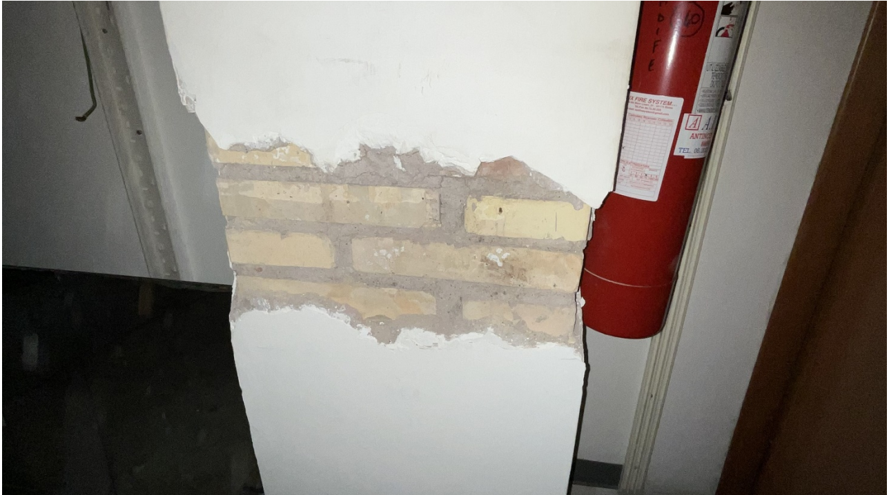
Pilastro in mattoni piano +1.26
