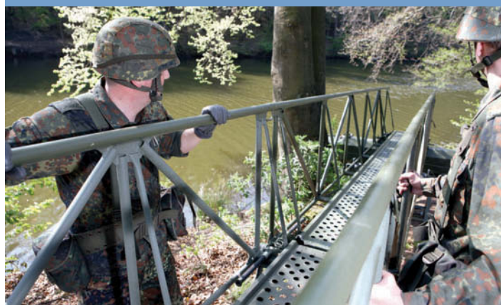
Launching the First Modules
