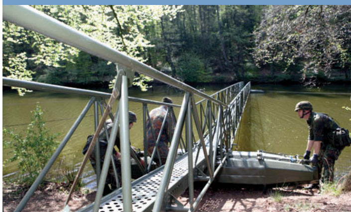
Bridge Extension with Float Support
