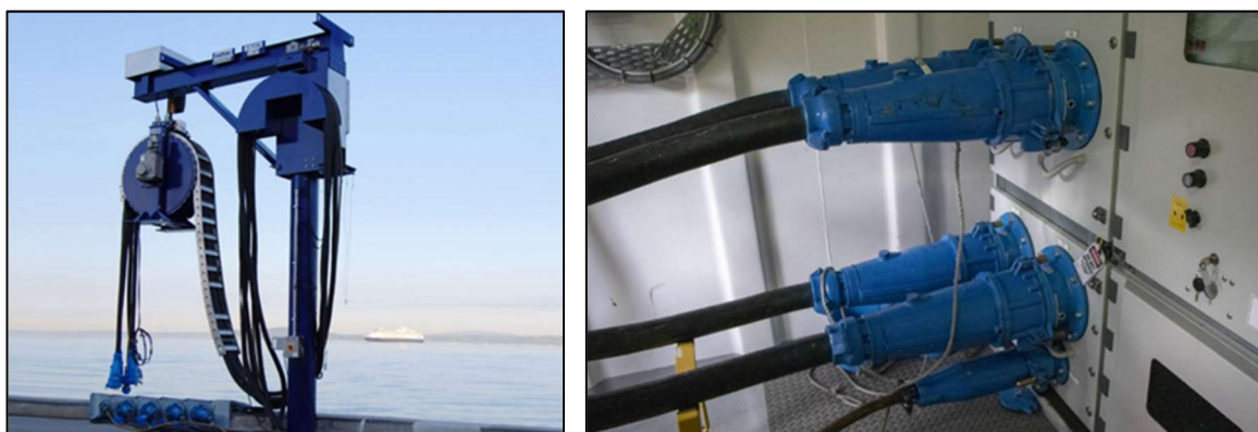
Figure 22 - Shore Connection System
