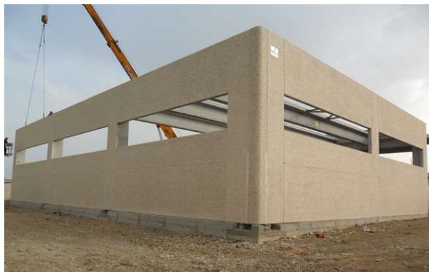
Figura 34 – Area logistica – Capannoni prefabbricati in c.a.
